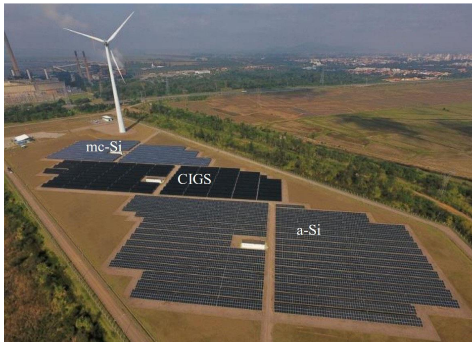
Figure 18: The ENGIE PV power plant "Cidade Azul" in Tubarão, with multi crystalline (mc-Si), CIGS and amorphous microcrystalline PV power blocks [15]
